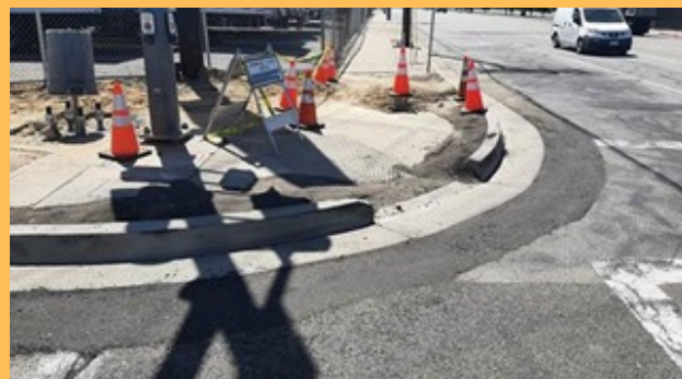
Road Repair Work At The Intersection of Mill and Arrowhead (Ward 3)
